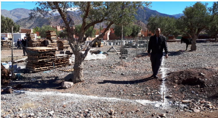
Chalking the area where house 6 will be built
